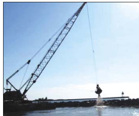
Dredging underway in Grand Marais Harbor, Minnesota.
